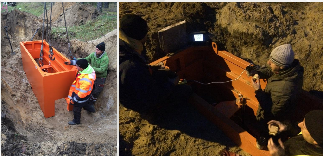
Successful pilot drilling and pulling a 220 mm reamer + 160 mm PE pipe in hard sand.
