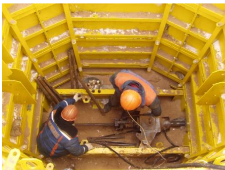
MNB-50 machine used for installing and replacing pipes under roads, with trench box and with modular shoring system.
