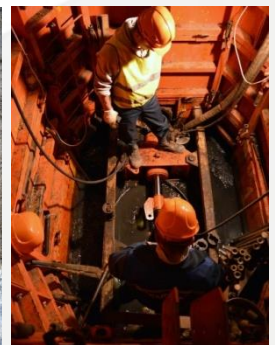
MNB-50 machine used for installing and replacing pipes under roads, with trench box and with modular shoring system.
