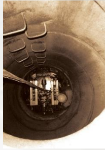
Assembly for working inside 1500 mm wells.
