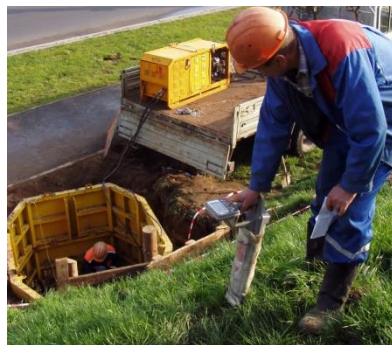
MNB-50 machine used for installing and replacing pipes under roads, with trench box and with modular shoring system.
